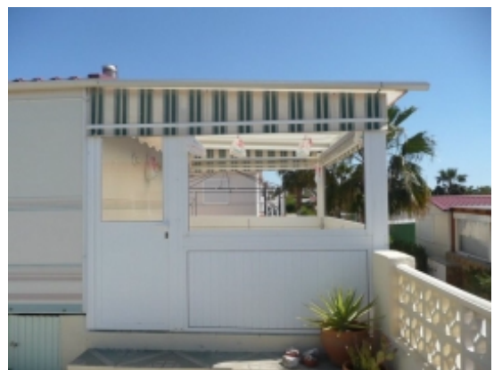
Exterior end conservatory
