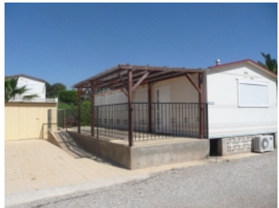
Raised patio and front of the mobile
